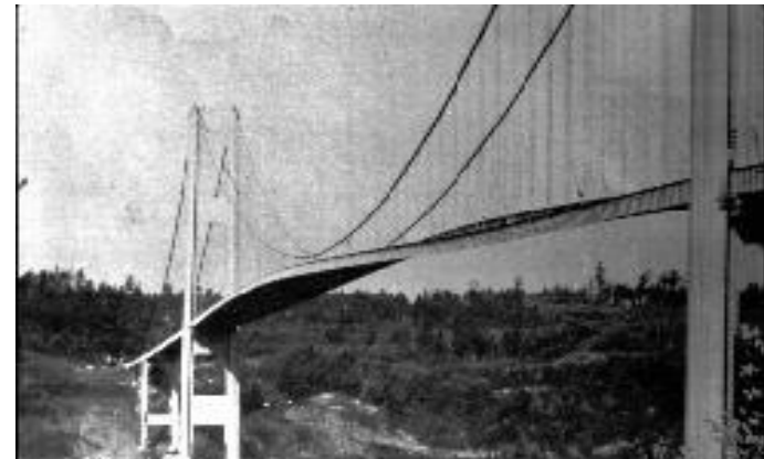
Figure 8.14 Takoma bridge (Washington) fallen down by "weak" wind 7th of November, 1940.
